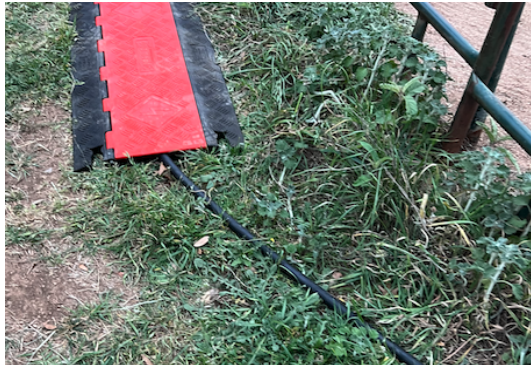
Image 5 - 10 Gauge DC Power Cables
